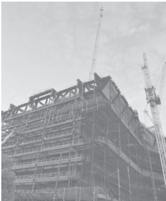
Figure 7: Even Google’s Kings Cross campus is taking 4+ years to construct.
